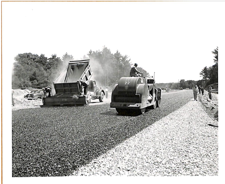
Bituminous Asphalt Mix on Newburyport Turnpike, 6/1952. National Archives Identifier 169136966
